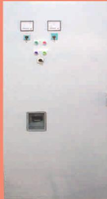
Soft starter is an advanced method of starting electrical motors by application of electronic devices like micro processor, SCR / Thyristor etc., and provides numerous advantages over other types of starters. In this panel voltage reduction and other vital features like controlled acceleration of motor are achieved by triggering SCRs at the desired firing angle by microprocessor. Once triggered the SCR allows current in one direction and turns off at zero current.
